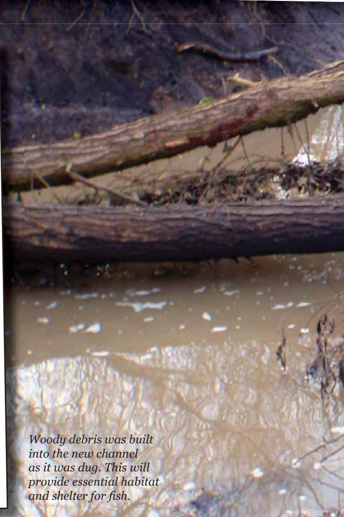
An old tree stump at the end of the new channel was used to create a small island and woody debris as shelter for small fish.
