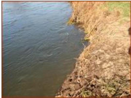
Heavy bank erosion where balsam has died off
