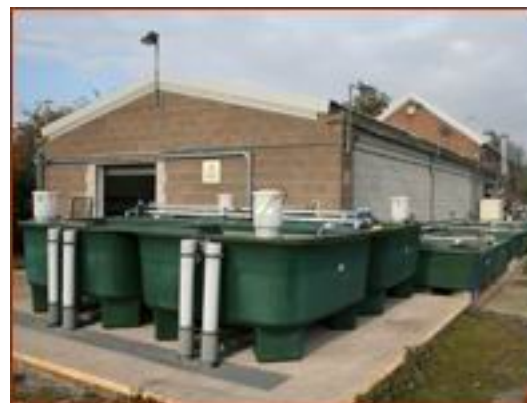
Just a few of Calverton`s holding tanks
