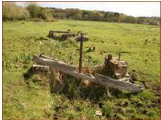
Nice old sluices, now high and dry
