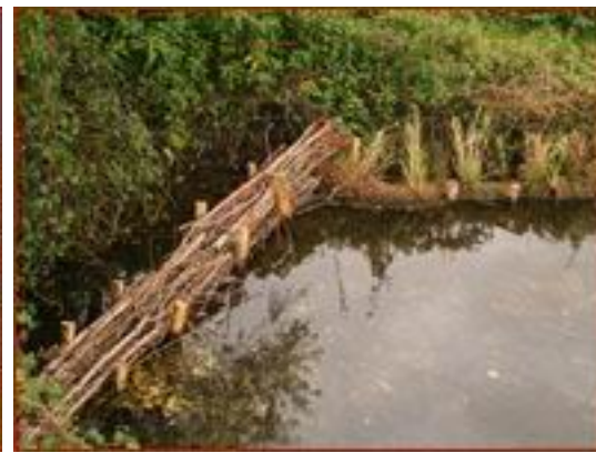
River repairs on the Wylfe, paid for by WSRT
