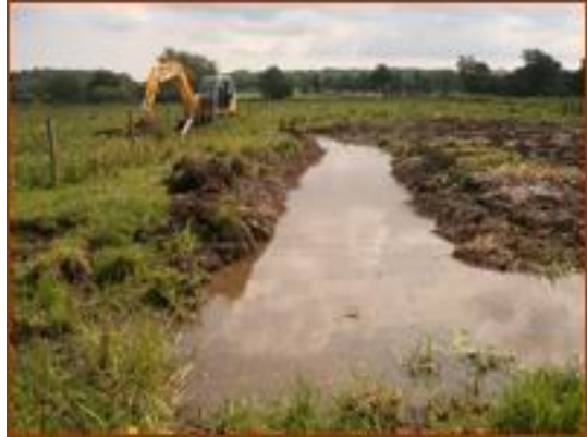
New fry bays nearly complete
