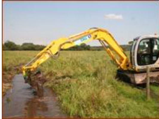
Years of silt being removed
