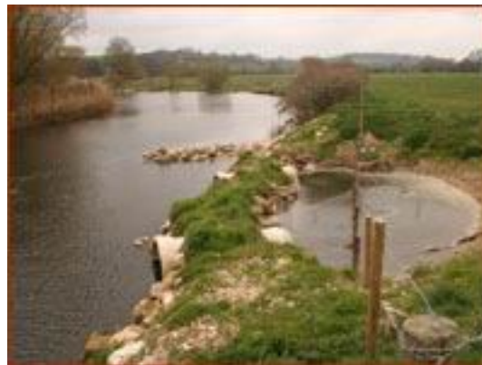
Fish refuge constructed just downstream of croy
