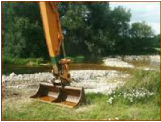
Repair of weir underway
