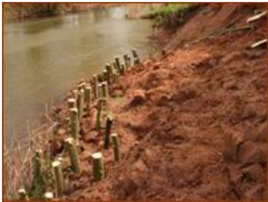
Collapsing and eroding bank, two years earlier
