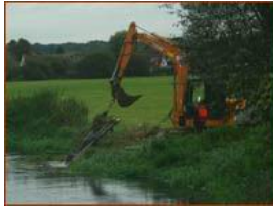
At last, the piles are out!
