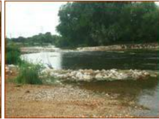
Reprofiled weir, narrowing river and scouring gravels
